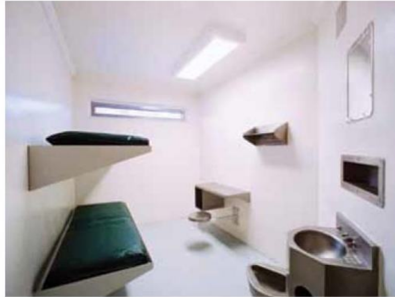
Fig. 1.2.18 Box module cells are often supplied with electric conduit and boxes, furniture, window and door embedments, and mechanical and plumbing chases cast in, reducing costly field work.
