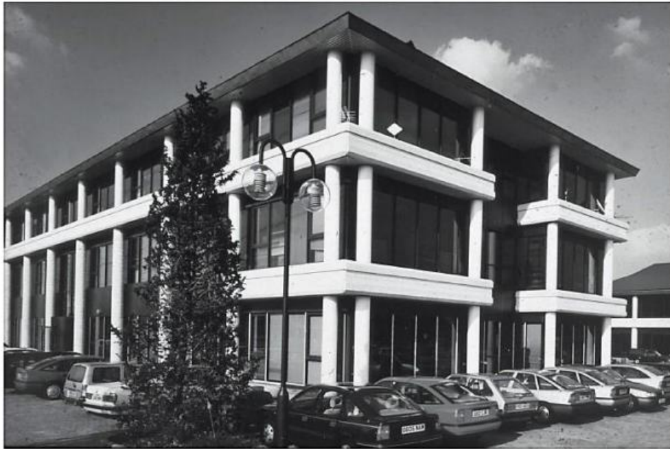
Precast 'skeletal' structure with integrated architectural columns and spandrel beams, Reading Business Park. (Courtesy of Trent Concrete Ltd., UK.)
