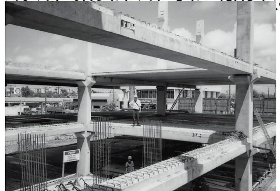
Precast concrete 'skeletal' known as 'semi-rigid' frame, Recife University, Brazil.
